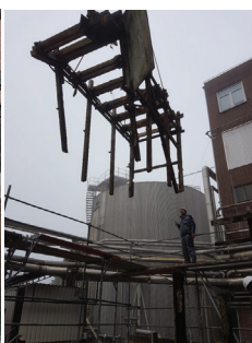
Dismantling of the old wooden structure.
