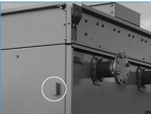
Detail male rigging guides on coil section
