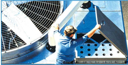
Hot water basin and optional distribution pan covers
