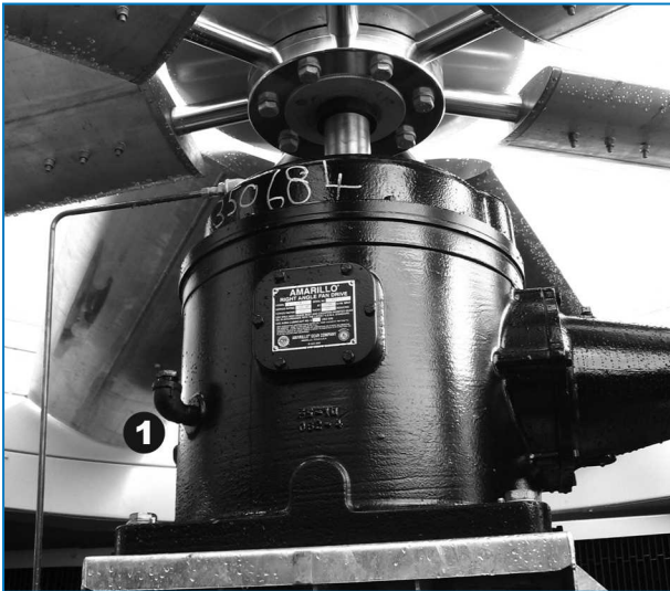
Single reduction gear drive
