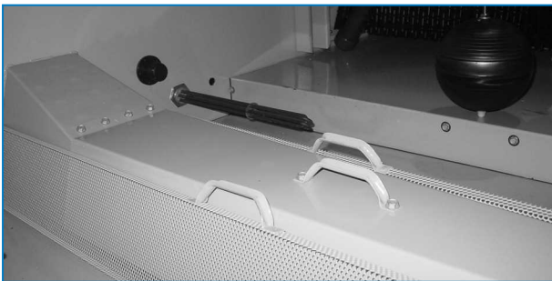
Cold water basin and basin strainer
