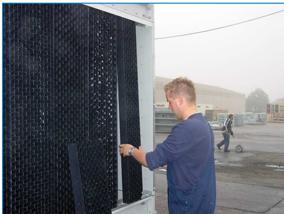
Remove combined inlet shields
