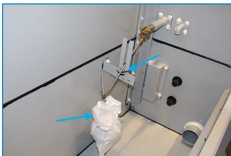
Fixation and wrapping of float ball
