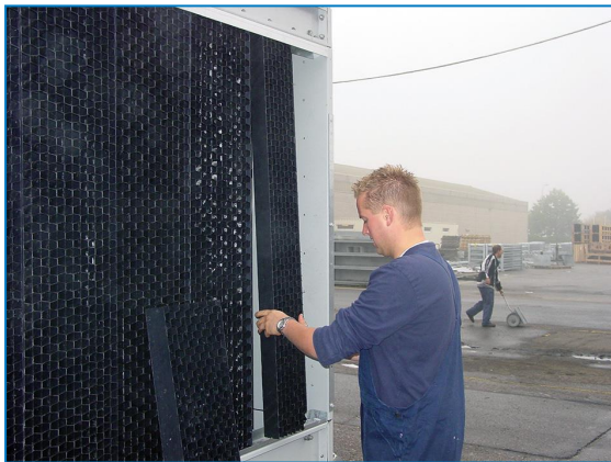
Remove combined inlet shields
