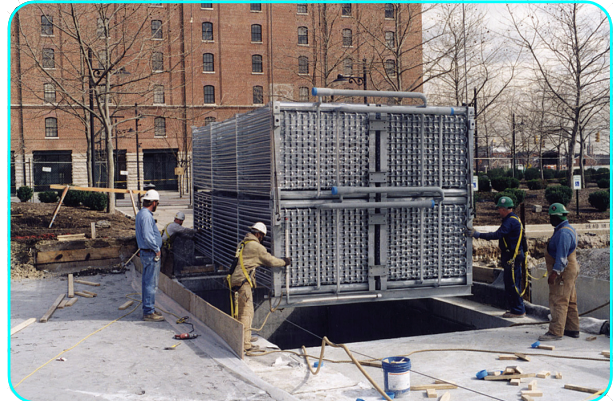
Installation of Coil Module
