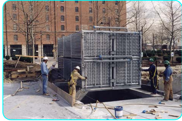
Installation of Coil Module
