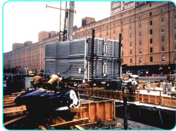
Coils installed in Concrete Tank
