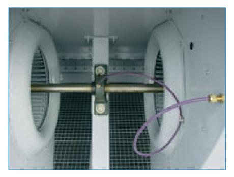
Extended lubrication lines with grease fittings can be used to lubricate fan shaft bearings. The fittings are located inside the plenum area next to the access door.
