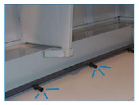
A sump sweeper piping system **increases water circulation and agitation** in the basin and is designed to be used in combination with a <u>filtration system</u>. It does all this:
