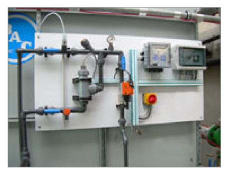
BAC offers a wide range of **automatic water treatment packages** to control corrosion, scaling, fouling and microbiological growth in cooling systems incorporating BAC condenser.
