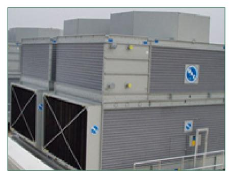
CXV-D condensers use **quiet and low kW axial fans**, but to reduce noise even further, you can extend your CXV-D condensers with <u>sound attenuation</u>:
