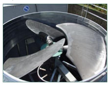
**Quiet and economical kW axial fans** mean CXV-D condensers make little sound. To reduce noise still further, choose the **Whisper quiet fan** alternative targeting optimal noise-reduction, with an aluminum hinged-blade design and unique end caps.
